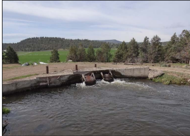
Photo 1: Southern end of Horsely Canal facing south
